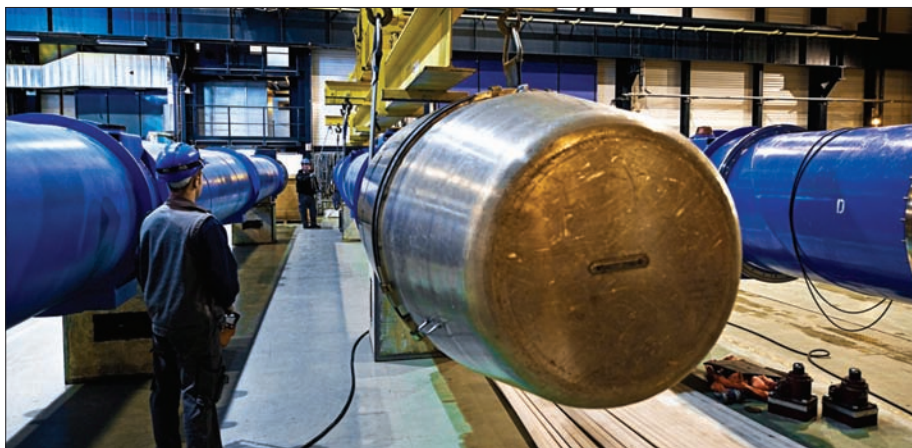
Replacement dipoles for sector 3-4 of the LHC are prepared for lowering into the tunnel.
