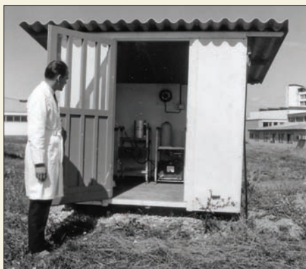
One of the four permanent radiation-monitoring stations installed on site.
